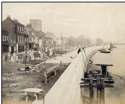
Embankment Under Construction, 1873. Photo: James Hedderley. Image courtesy RBK&C Archives.
