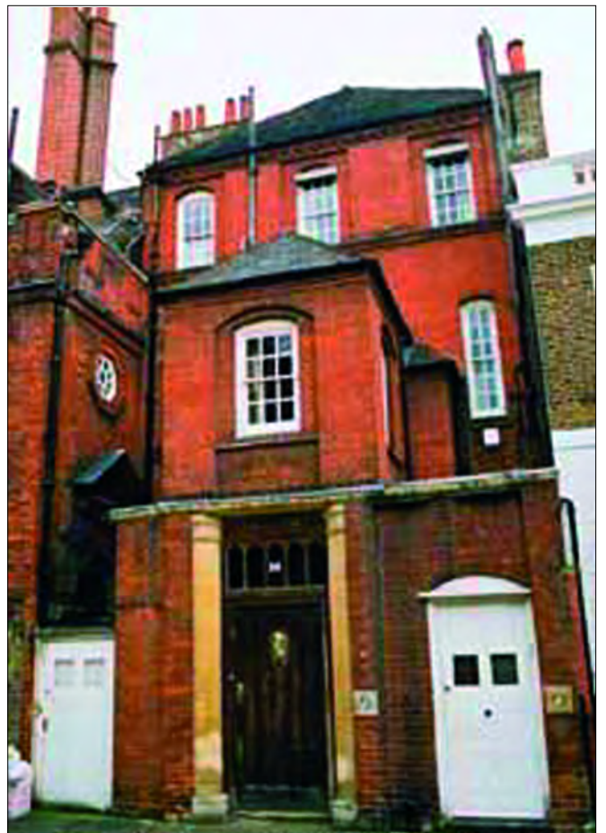
West House front
